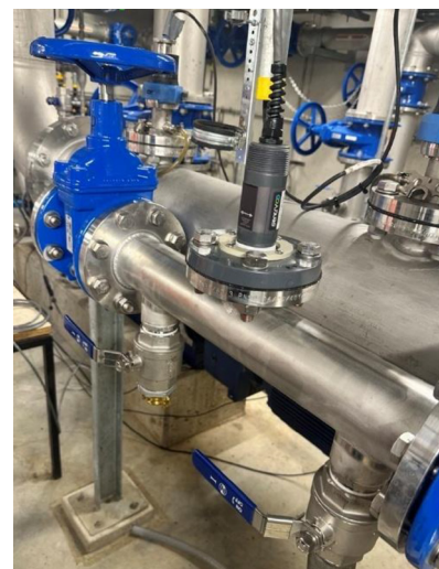
Figure 1: A SENTRY real-time VFA monitoring sensor installed on the recirculation line of the Ephyra digester.
